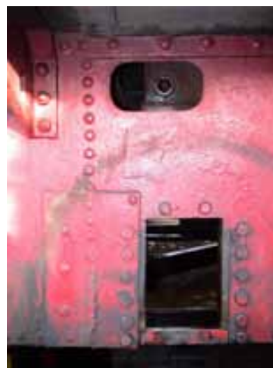
Scheurvorming scheenpoort links
